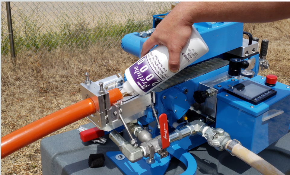
Prelubricating conduit prior to blowing fiber optic
